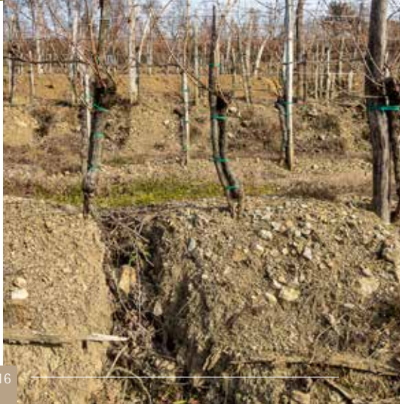
Figure 9: Erosion on terraces (photo by Borut Vrščaj).
