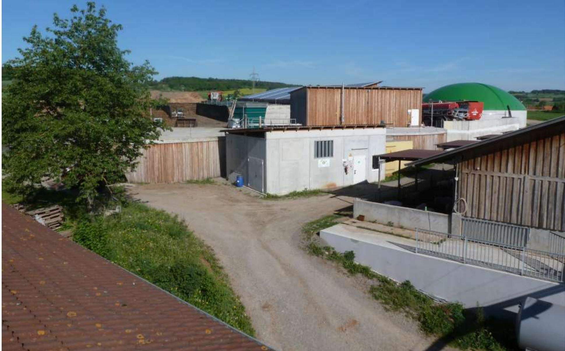
Gas storage (green part) 900 cbm, Liquid Fraction storage 2200 cbm (grey Part) plus 1000 cbm old storage, so 3200 cbm = 9 months of storage time
