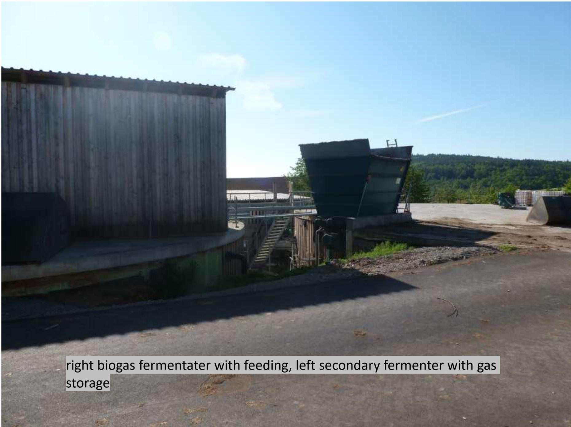
right biogas fermentater with feeding, left secondary fermenter with gas storage
