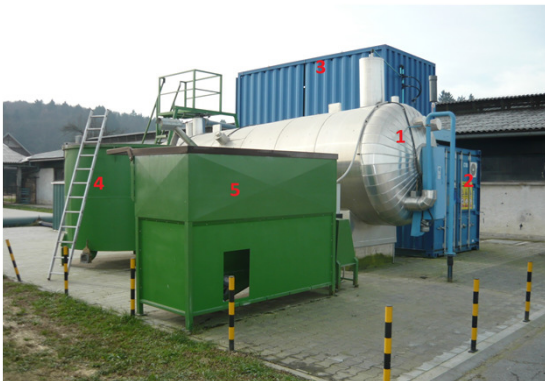
Picture: Parts of modular micro biogas plant: 1 – digester, 2 – energetic container with units for: processing of input substrate, cleaning of biogas (first stage), biogas powered cogeneration (electrical and thermal energy production), thermal energy storage and electronic regulation of process of biogas production, 3 – biogas holder integrated in container for mechanical protection, 4 – hydrolysing unit for hydrolysis of solid biomass, 5 – dosing system for adding solid biomass connected with milling unit for mechanical preprocessing of solid biomass with milling.
